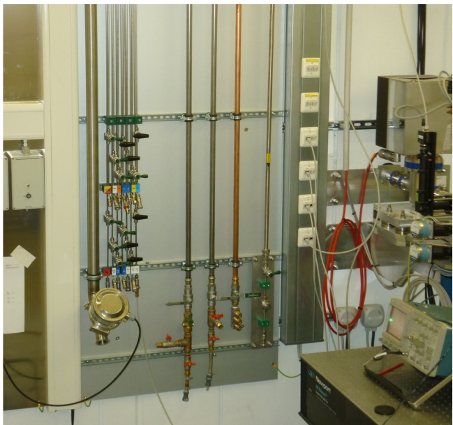
Gas supply for toxic, flammable and inert gases at beamline P65
